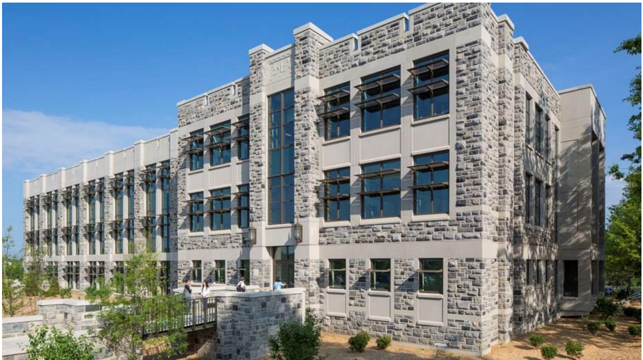
Human and Agricultural Biosciences Building 1 (HABB1), completed in 2014 for graduate students, faculty and laboratories of the BSE and Food Sciences and Technology Departments.
