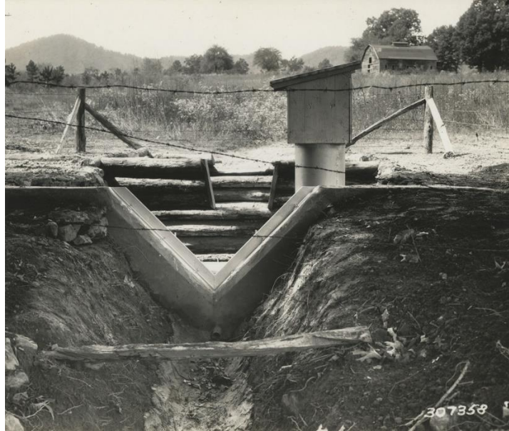
Weir/flume combination used in Soil and Water Conservation research in the Dust Bowl/Great Depression era.
