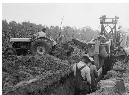
Tile drain installation, late 1910s
